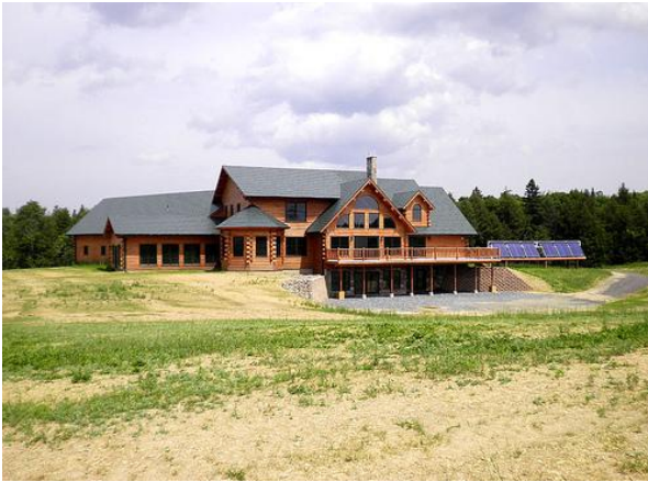
An example of a home manufactured by Katahdin Cedar Log Homes in Oakfield
